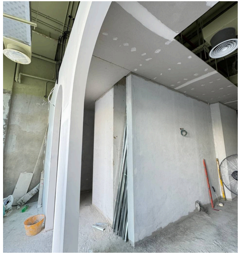
VALERI PILATES STUDIO ARJAN UNDER CONSTRUCTION
